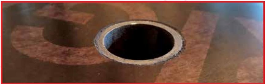
“Steel rings around the tie-rod holes provide to very good protection for plywood”
